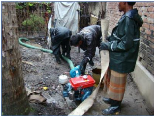
(c) Diesel pump
