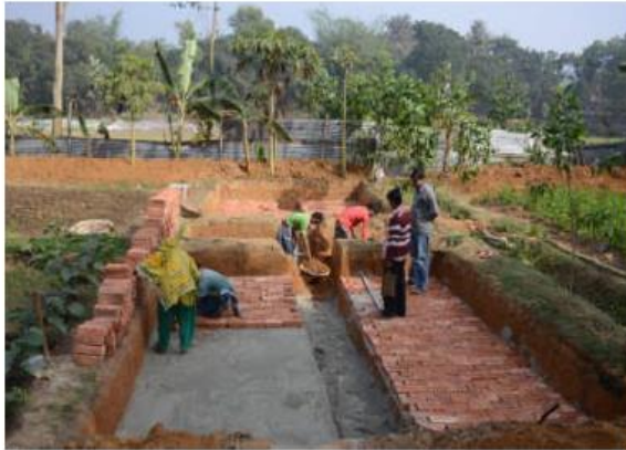
(a) Drying beds – masonry work
