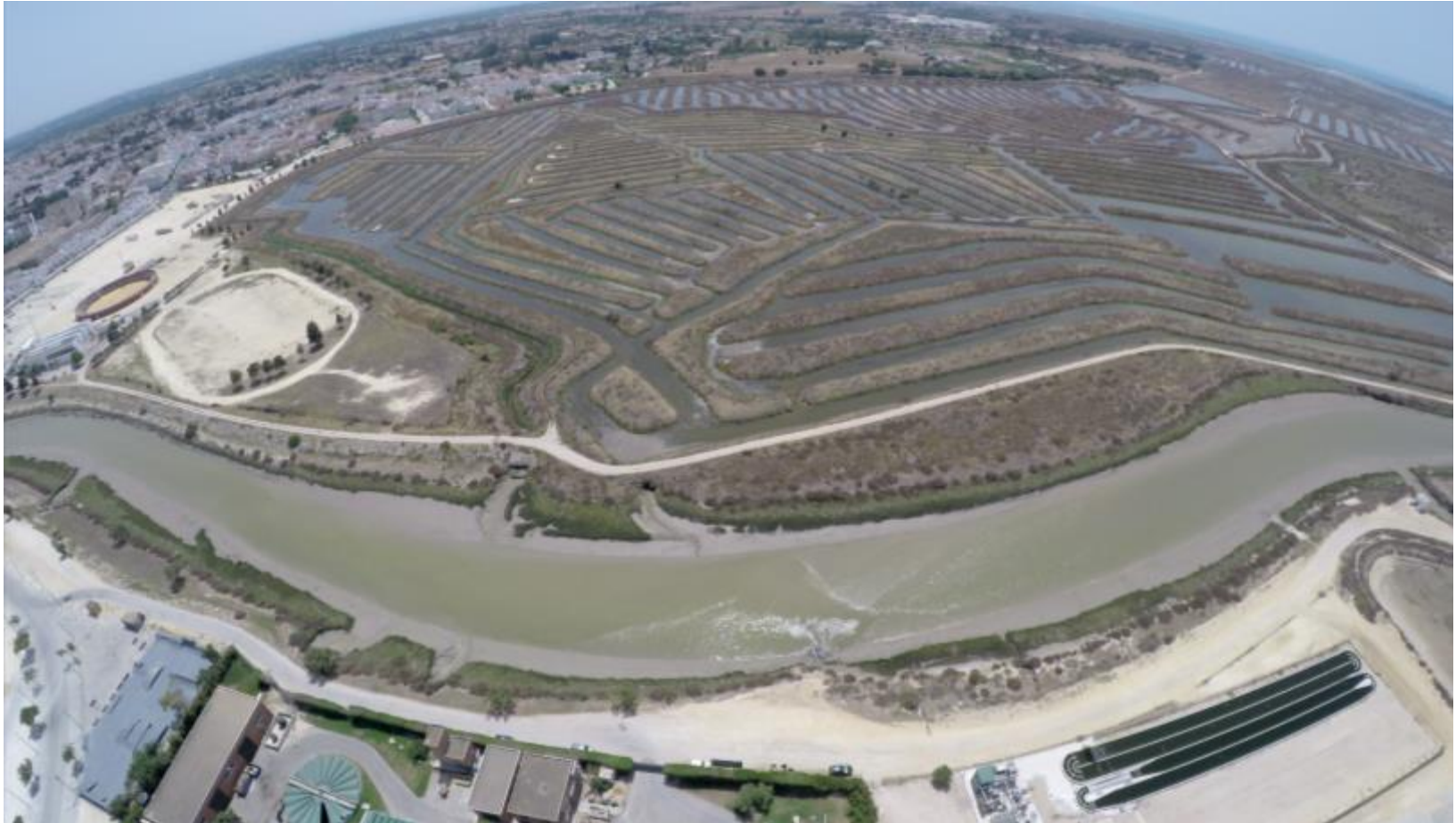
All-gas project, FCC Aqualia
