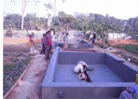
(b) Drying beds – plastering work
