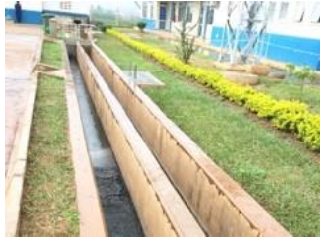
Grit removal + Parshall flume
